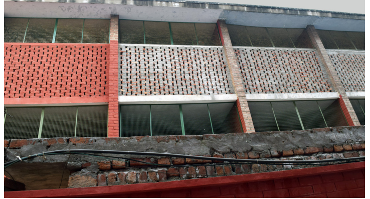
The exterior is also still in need of completion
