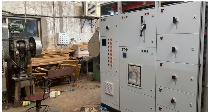
New electrical panels being installed.
