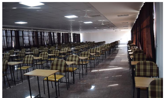
Renovated & installed air-conditioning for Exam Hall
