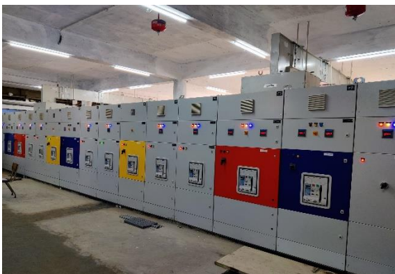
Installed 3 new generator sets in the Electrical Substation
